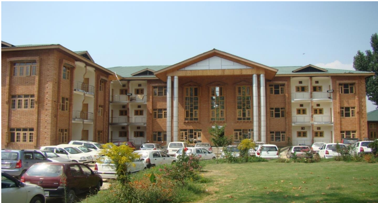
Hostel Block at IMPARD Main Campus, M. A. Road, Srinagar
