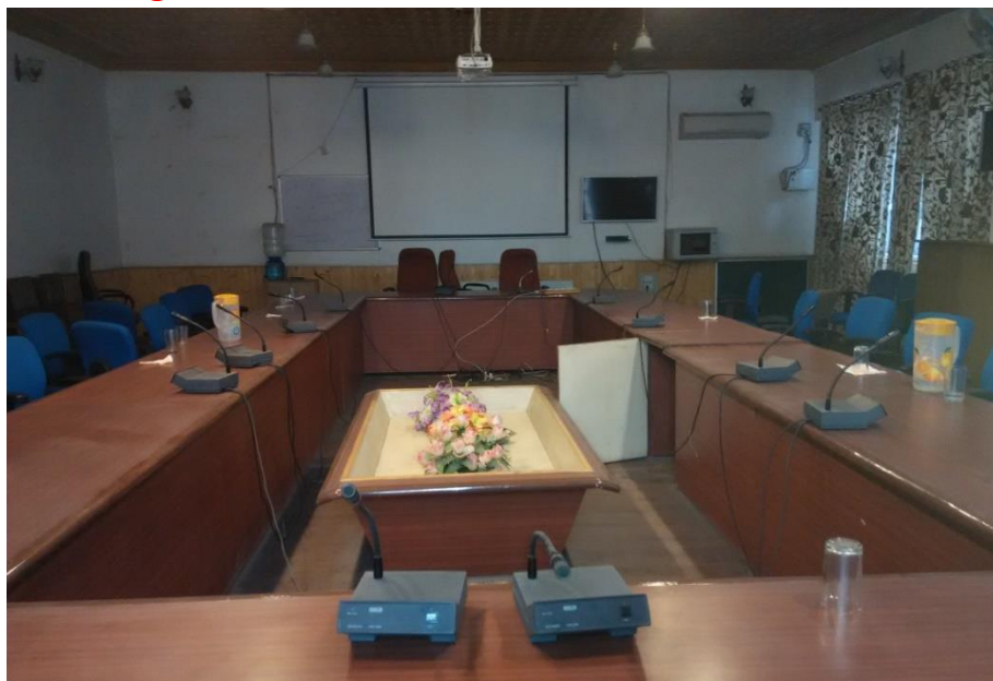
Video Conferencing facility installed at IMPARD Main Campus, M. A. Road, Srinagar
