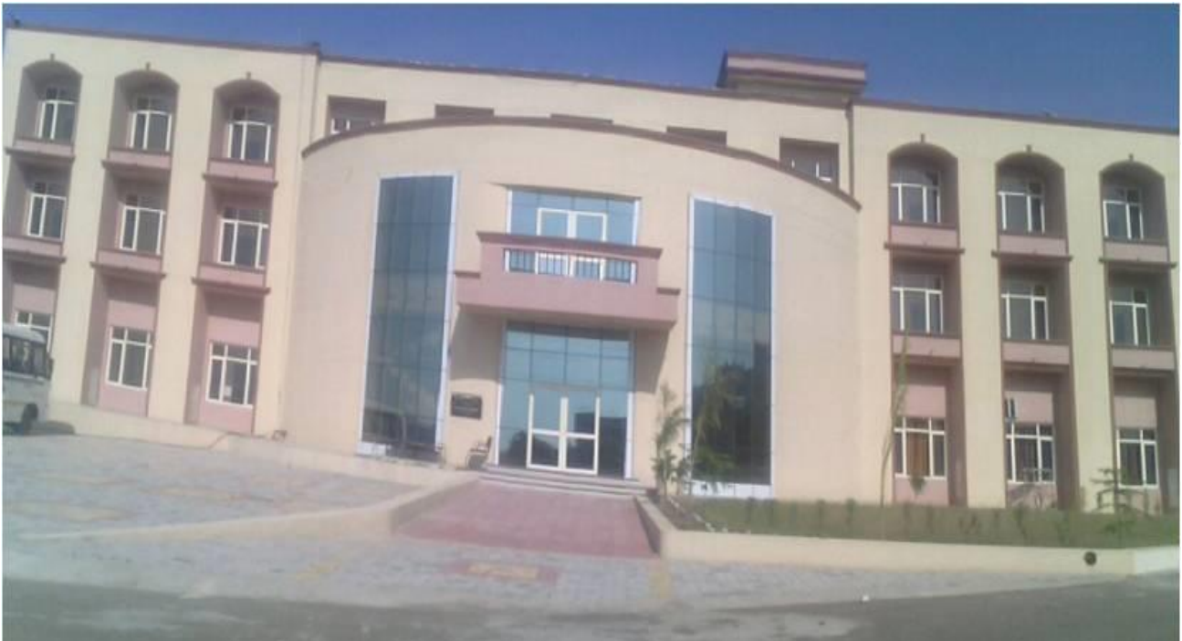
Hostel Block at IMPARD Regional Centre, Sidhra, Jammu
