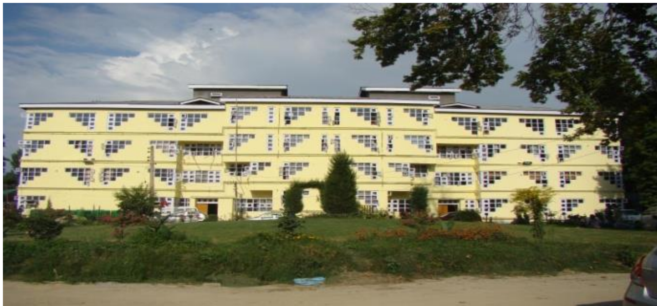
Administrative-cum-Academic Block at IMPARD Main Campus, M. A. Road, Srinagar
